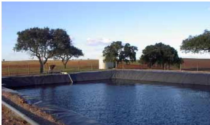
Fig. 14. Wastewater treatment system at Mingorra
